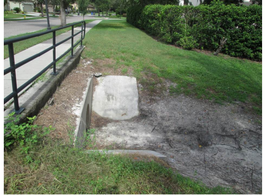
North side of culvert crossing on Hampton Lake Drive
