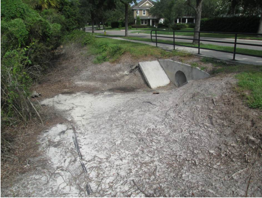
South side of culvert crossing on Hampton Lake Drive
