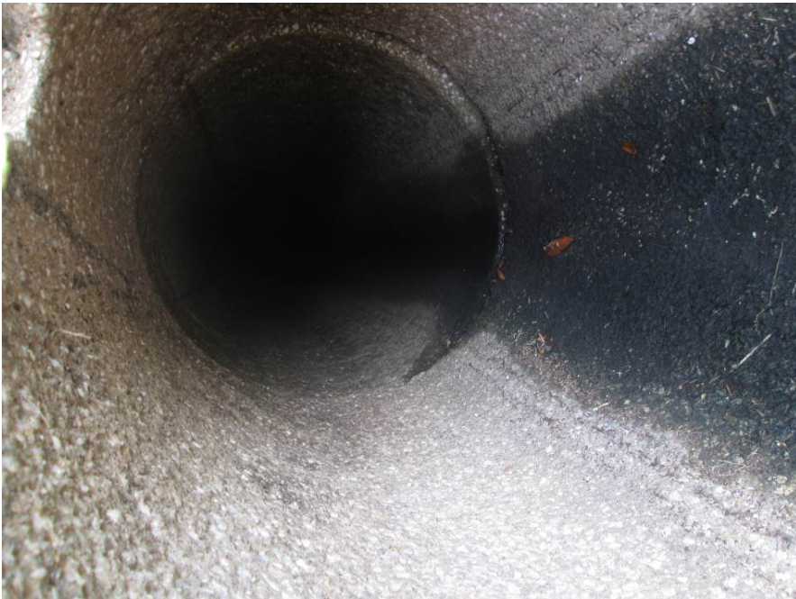
Pond 8 – MES end dropped slightly, void above joint
