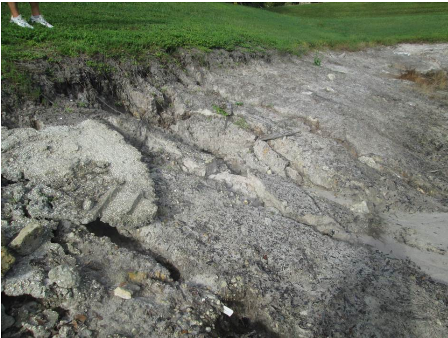
Pond 38 – erosion on south side (from Fire Hydrant discharge?)
