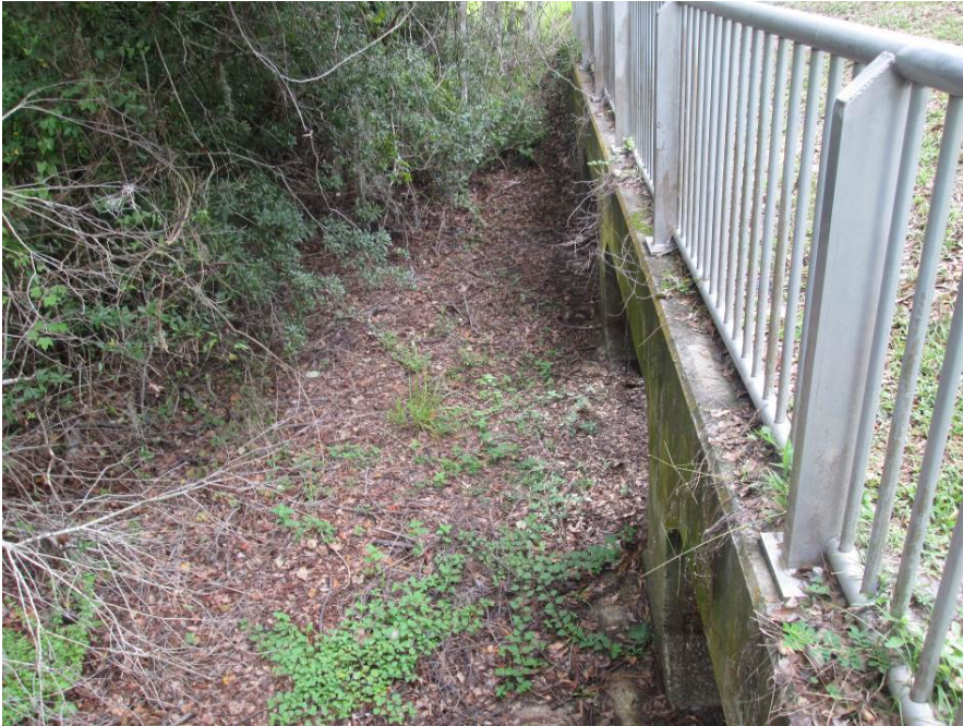
East side of culvert crossing on Heron Crossing Drive
