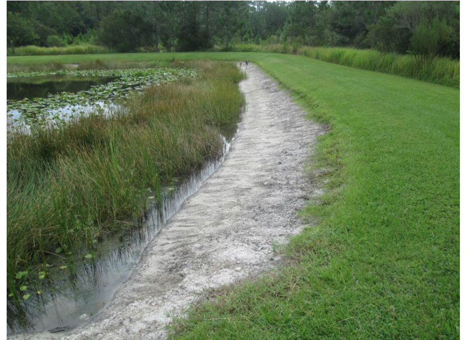
Pond 32 – Southwest corner of pond viewing east
