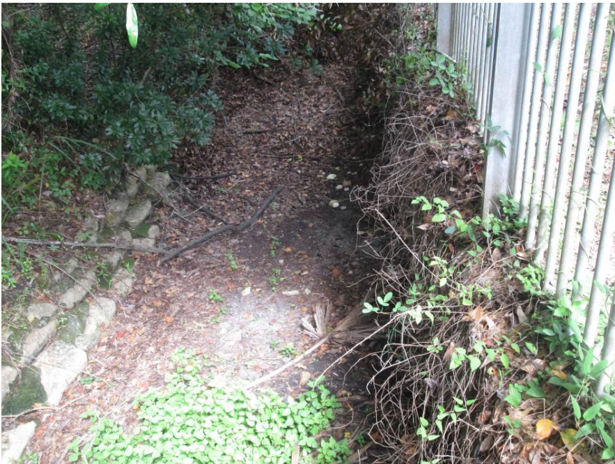
West side of culvert crossing on Heron Crossing Drive
