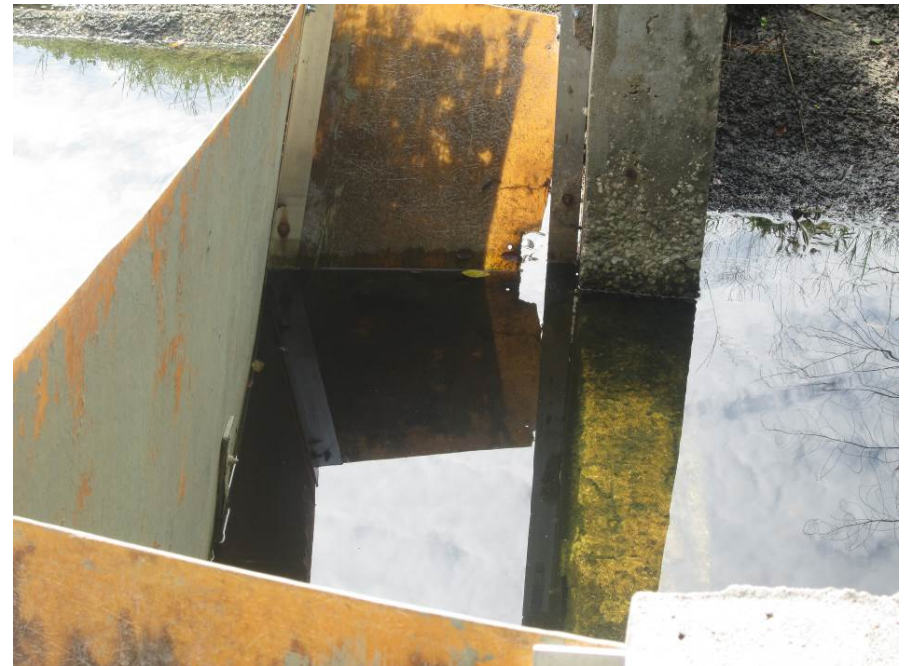
Pond 16 – Remove broken fiberglass skimmer, replace with aluminum one
